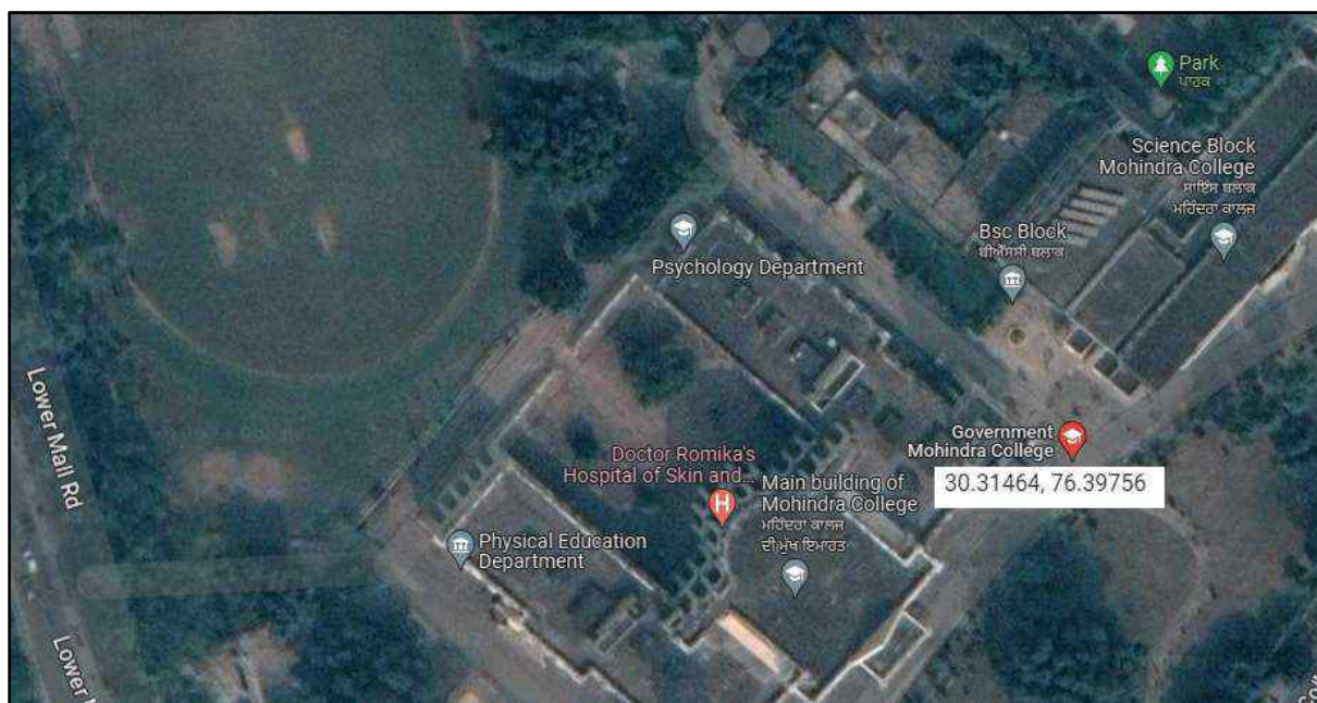
Figure 1: Aerial view of the Government Mohindra College, Patiala
