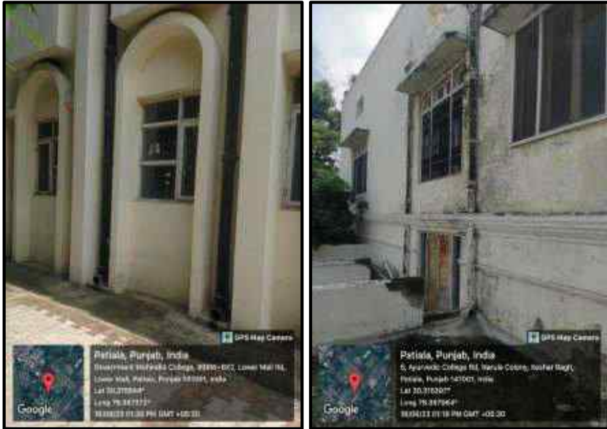
Pipes connecting from Rooftop to ground (Manhole and lawns) Photograph of Rain Water Collection Pits
