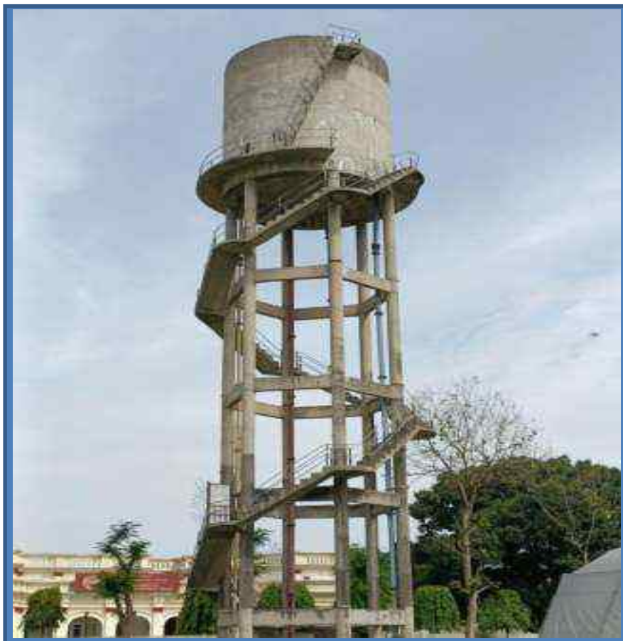
Water Storage Tank
