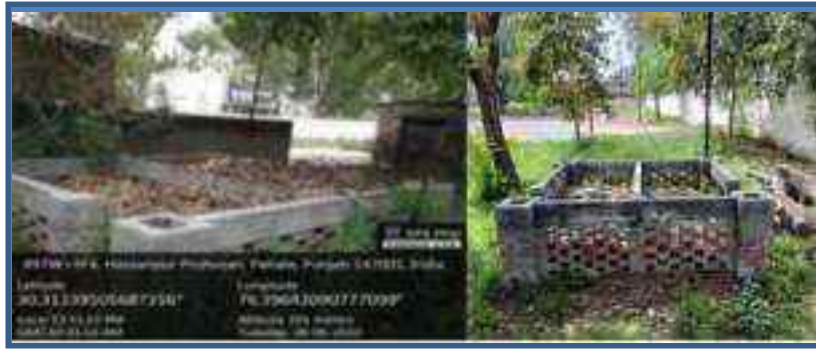
Composite pit near gate no. 3
