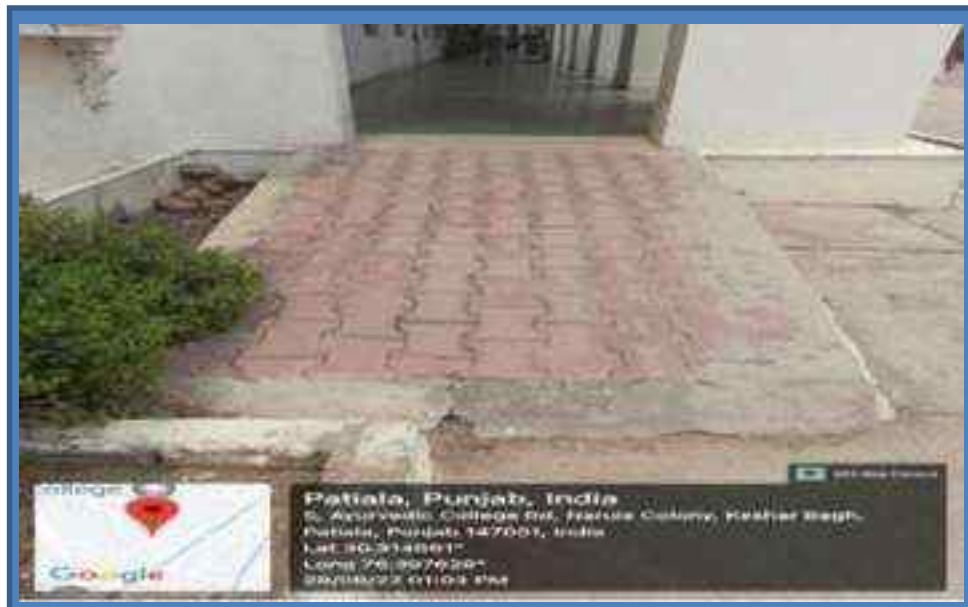
Ramp at Science Block Entry Point
