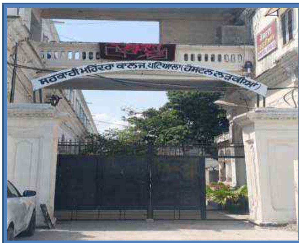
Signage at Girls Hostel Entrance
