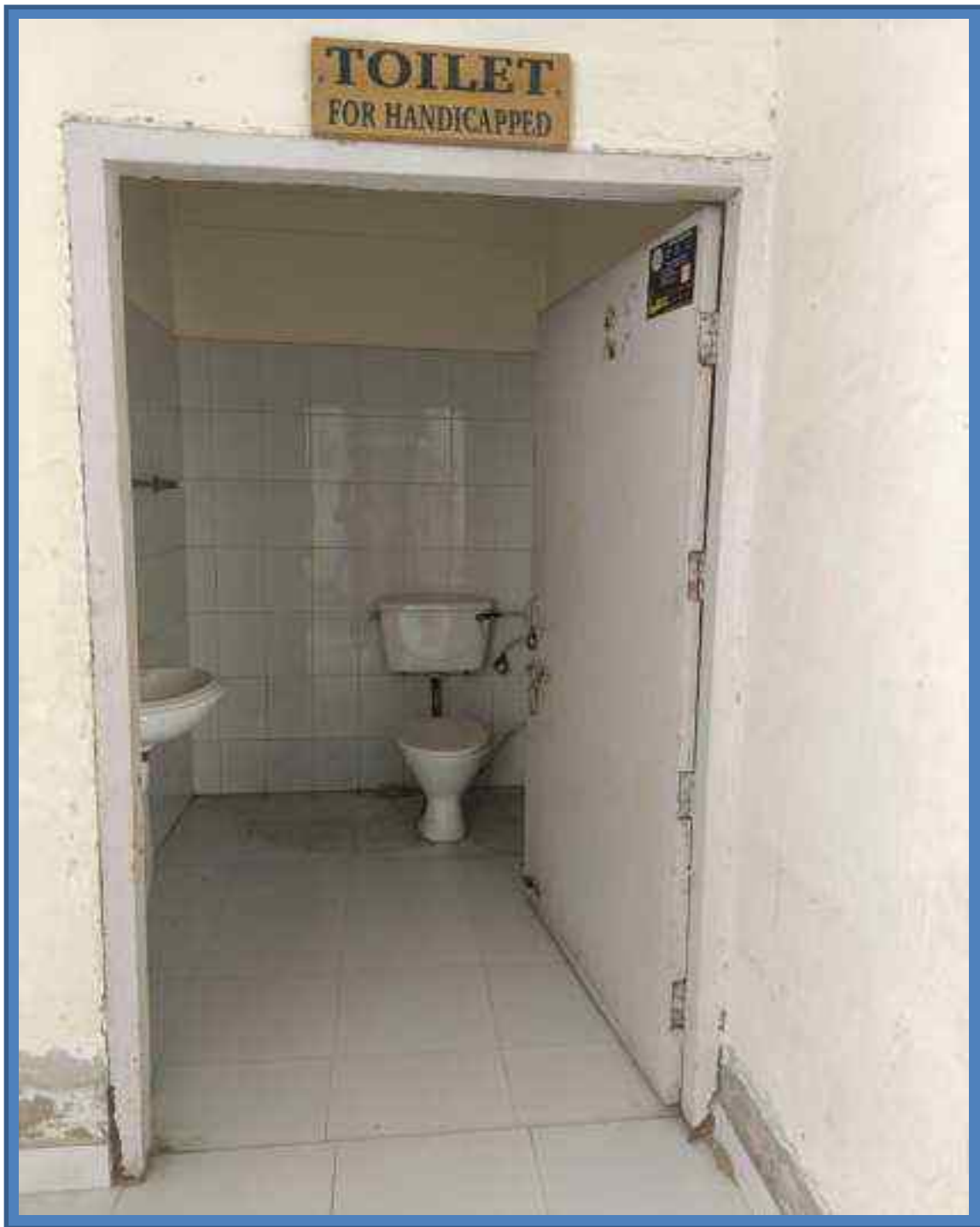
Washroom facility for Handicapped
